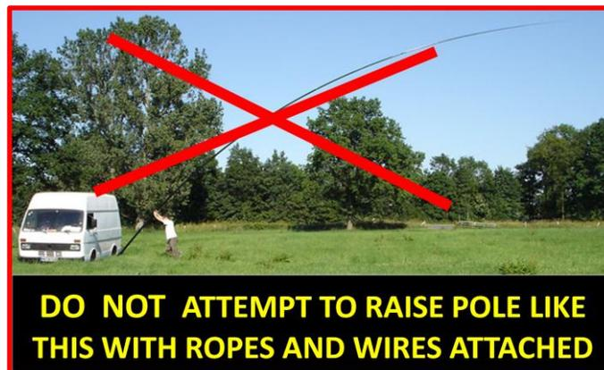
**PLEASE ERECT THE POLE ONE TIME WITHOUT ANY WIRES ATTACHED.**
